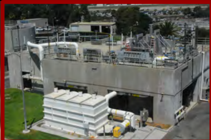
Step 1 Preliminary Treatment: Removes the very large and heavy contaminants.
