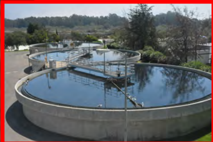
Step 2 Primary Clarifiers: Remove floatable and settleable solids
