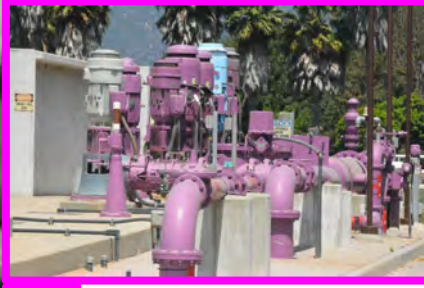
Step 7 Reclamation: Coagulation, flocculation, filtration, and disinfection before reuse for irrigation.
