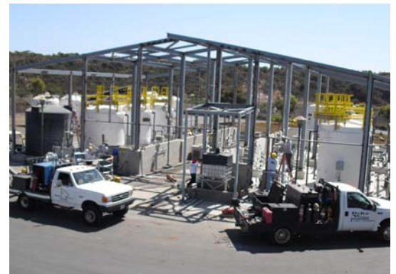
New Chemical Containment area shown under construction.
