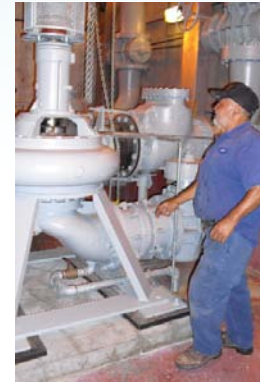
Installation of new high-efficiency pumps.
