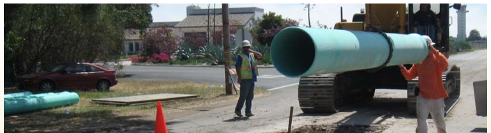
A new sewer pipeline is being built along Fairview Avenue.
