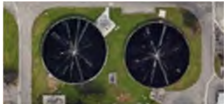
Biofilters at GSD (BOD removal)
