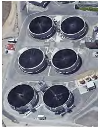
Nitrifying trickling filters at Truckee Meadows Water Reclamation Facility
