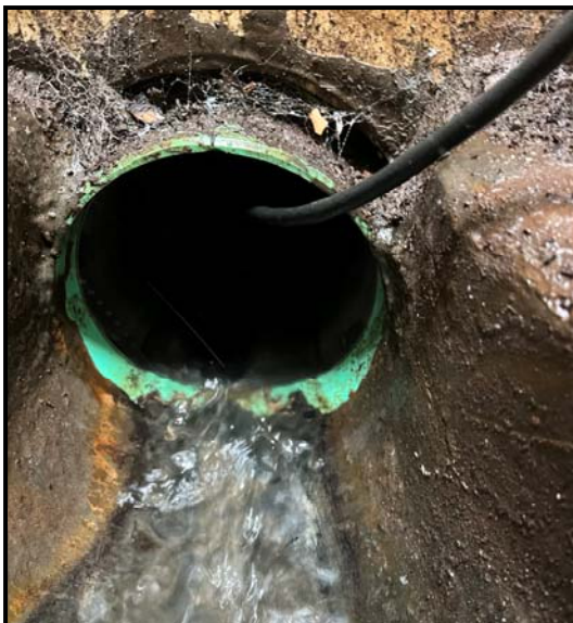
Meter installed inside of the MH Effluent line.
