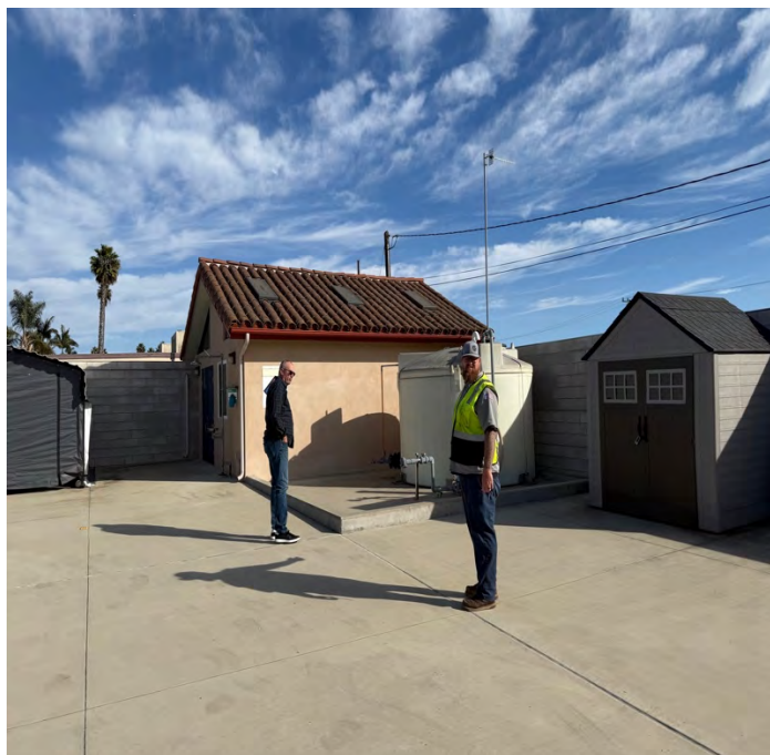
Photo 3: Station site overview
