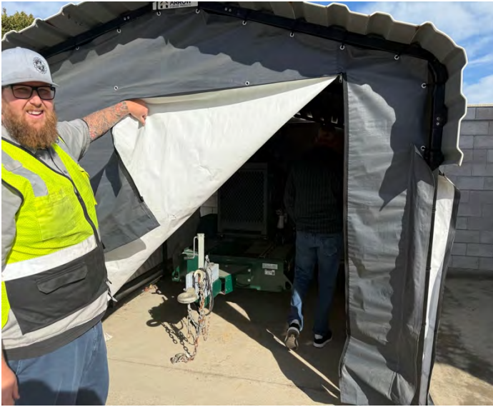
Photo 5: Inspection (station covered portable backup pump stored onsite)
