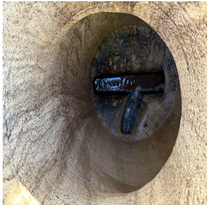
Photo 4: Inspection (FOG); no significant buildup of solids observed
