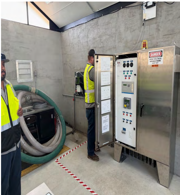
Photo 11: Inspection (station pump controls); station not monitored by collections operators on SCADA who rely on plant staff for readings
