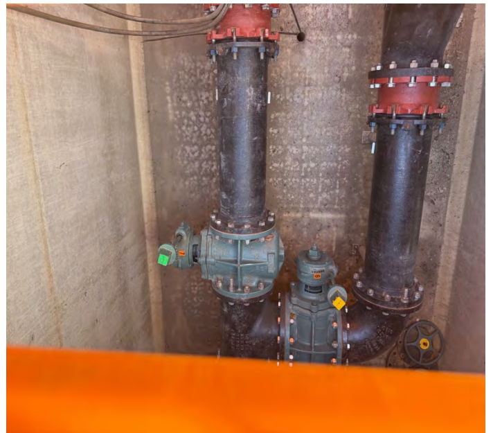
Photo 24: Inspection (force main valve pit)
