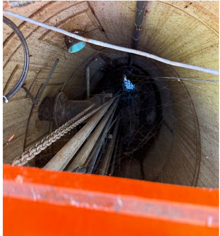
Photo 20: Inspection (station wet well with some plastic shampoo bottles from upstream hotel observed floating on mat)
