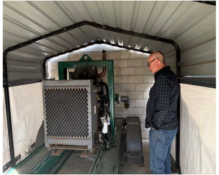
Photo 6: Inspection (station covered portable backup pump stored onsite)
