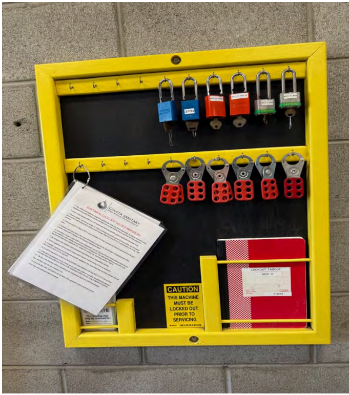
Photo 9: Inspection (lockout/tagout equipment)
