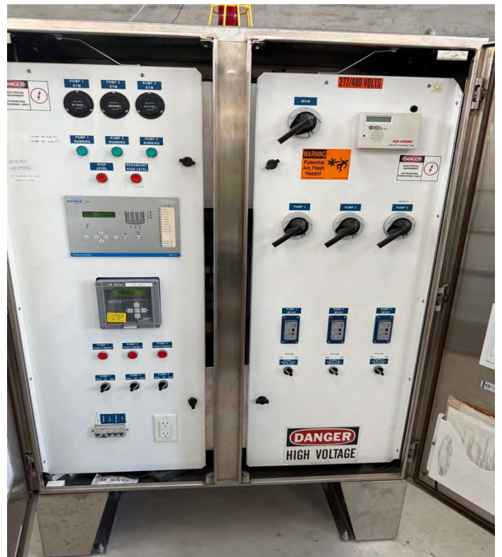
Photo 12: Inspection (station pump controls)
