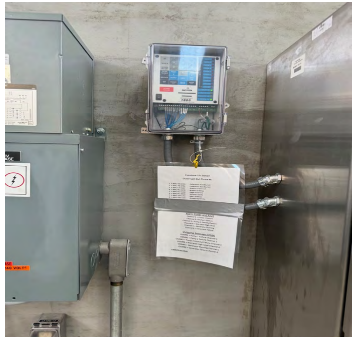
Photo 10: Inspection (station auto-dialer system)
