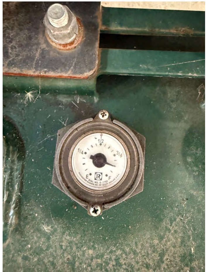
Photo 8: Inspection (station fuel tank level 3/4 + full)
