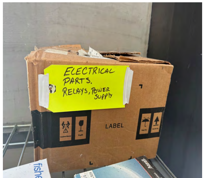
Photo 16: Inspection (station pump controls)
