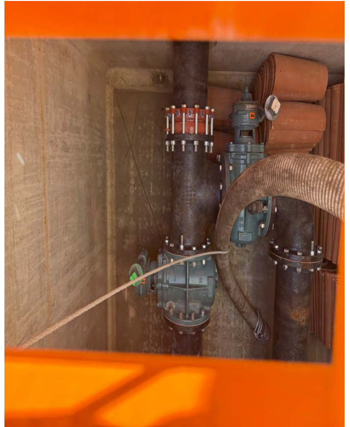
Photo 22: Inspection (force main valve pit)
