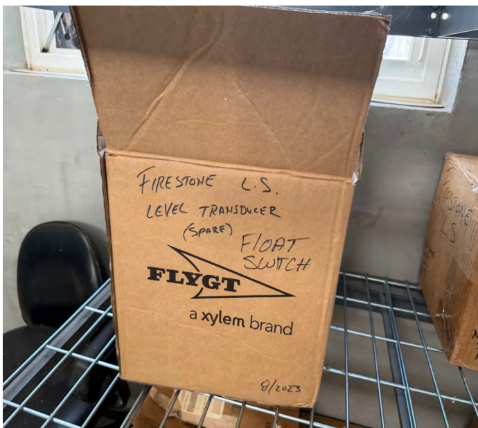
Photo 15: Inspection (station pump controls)
