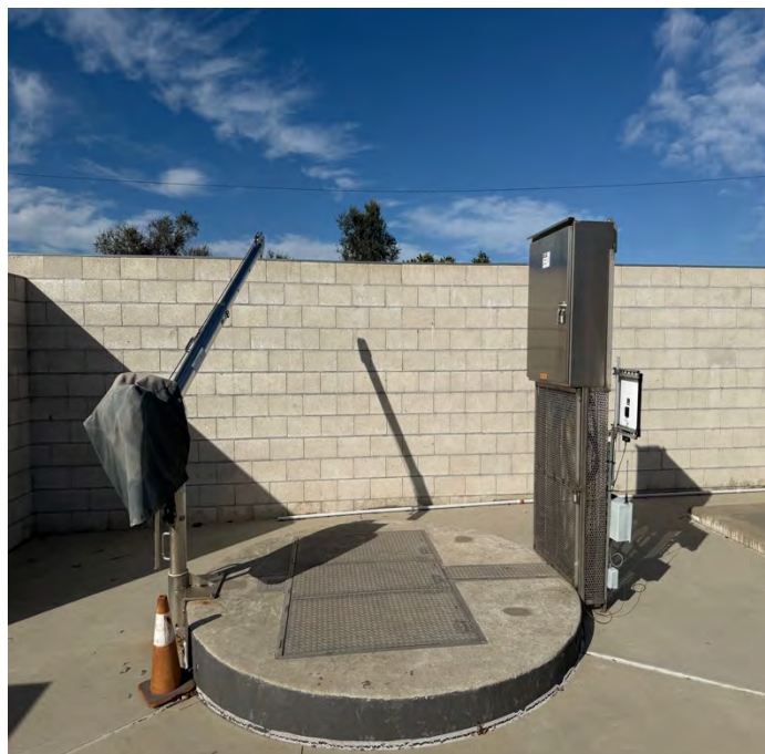
Photo 4: Inspection (pump pit/access with crane); no containment plan for station
