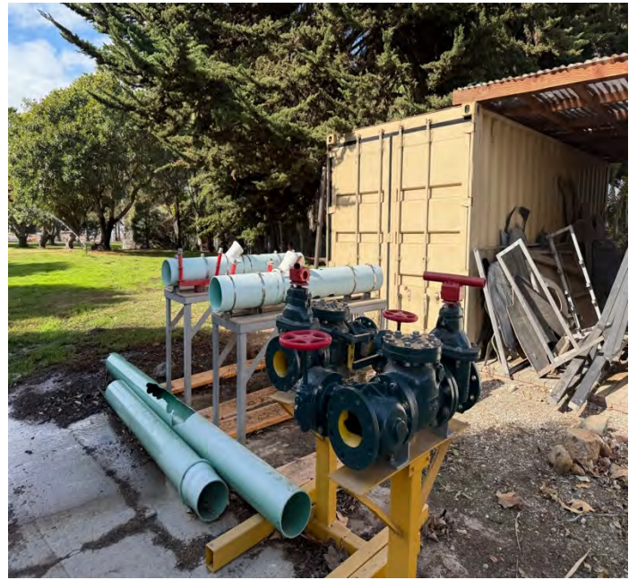
Photo 2: Inspection (training equipment, view 1)
