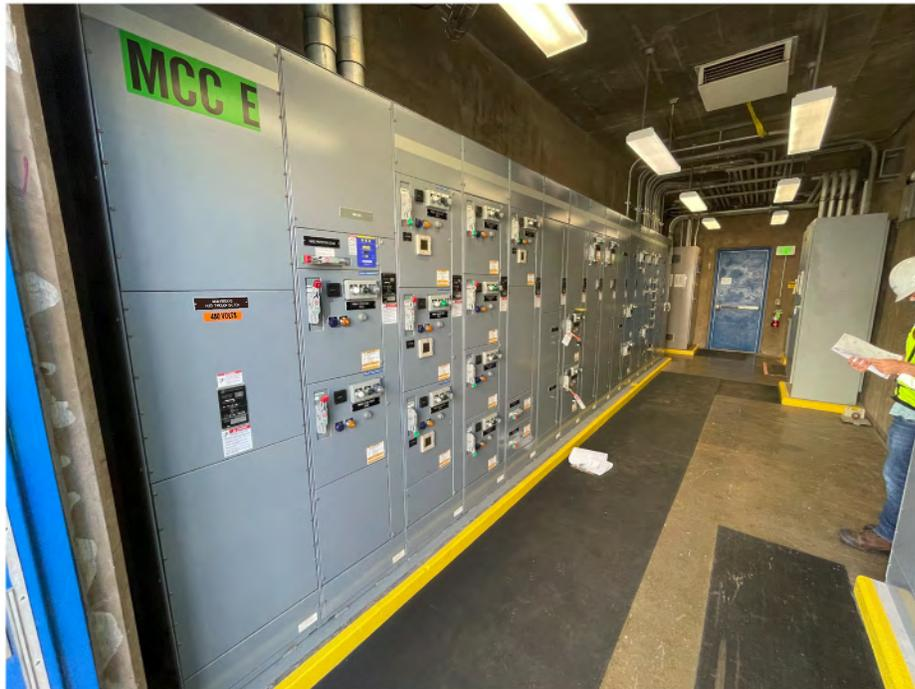
Figure 2-3. HSW receiving station electrical loads will be routed to headworks MCC-E (pictured above)
