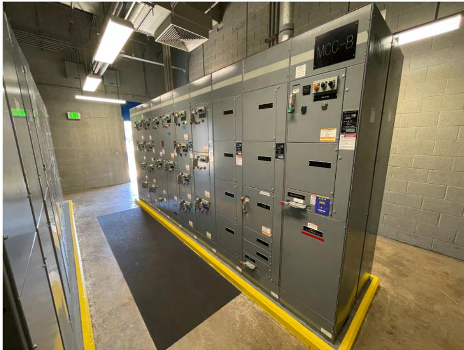
**Figure 3-8. Gas pretreatment system will be powered from Existing MCC-B (pictured above)**
