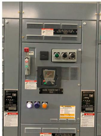
Figure 3-7. Existing sludge dewatering pump VFD to be replaced with new VFDs in existing bucket
