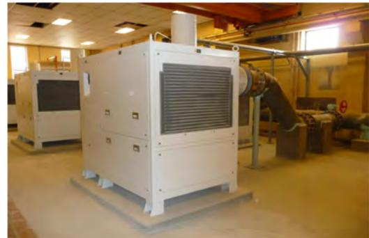
**Hazen replaced Rivanna's engine blowers with high speed turbo blowers and installed a 355KW CHP system to lower energy demands**
