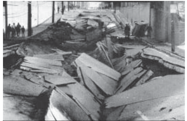
A safety issue: Discharges of hexane from an industry into Louisville, Kentucky's sewer system collapsed sewer lines and destroyed streets throughout the city in 1981.
