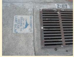
**STORM DRAINS** collect runoff and stormwater from streets, and discharge it untreated into the ocean.
