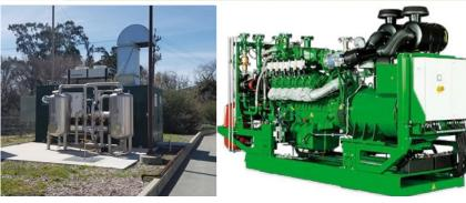
• A biogas pretreatment system to reduce hydrogen sulfide (H2S), siloxanes, and moisture in the digester gas used to fuel the CHP engine.
