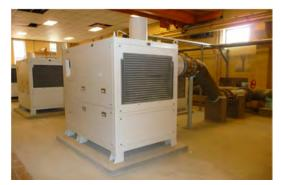
Hazen replaced Rivanna's engine blowers with high speed turbo blowers and installed a 355KW CHP system to lower energy demands
