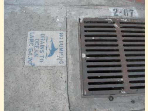
STORM DRAINS collect runoff and stormwater from streets, and discharge it untreated into the ocean.
