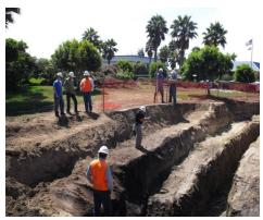
Trenching needed to satisfy requirements of a fault study for the wastewater treatment plant upgrade project. No fault lines were found clearing the way for construction on-site.
